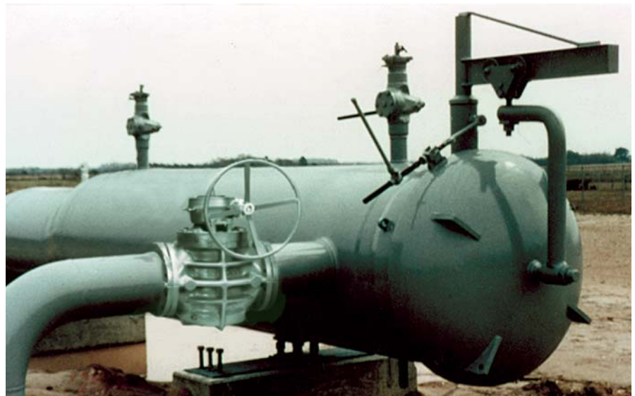
A Yale® Figure 500R™ Closure installed on pig launcher
